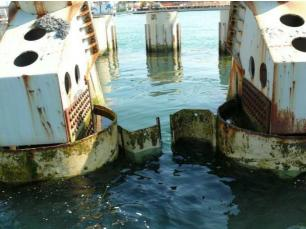
On 23<sup>rd</sup> June 2011, the ship "Haci Emine Ana" loaded with a cargo of wheat in bulk, during the manoeuvres aimed at entering into the port of Venice, because of a sudden failure of electrical ship control systems, collided with the outer side of the barrier (MOSE) placed on the south dike of Malamocco harbour entrance.
